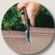
The panel can be cut using standard vinyl knife or cutter.
